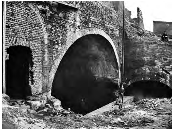
The Great Tunnel in the 1880s
